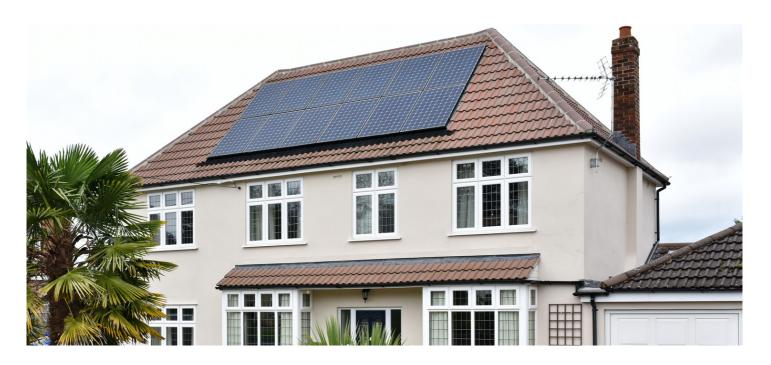
One solar panel typically consists of around 30 cells (those familiar-looking blue squares you often see in a solar panel). It can generate between 250-400W of power in full sunlight, depending on brightness, size of panel and other things like temperature. The panels generate a direct current of electricity, which then passes through an inverter to convert it into an alternating current. This generated electricity can then be exported into the National Grid or used in the home.
