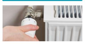
Control the heating effectively using the room thermostat, heating programmer/timer and thermostatic radiator valves:
